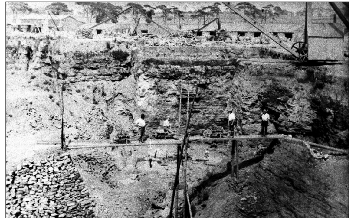
An interesting picture shows how the quarryman moved across the quarries by building piles of waste stone, which supported planks c1890. Note the fir trees growing in the background along the Stoke to Higher Odcombe road.
