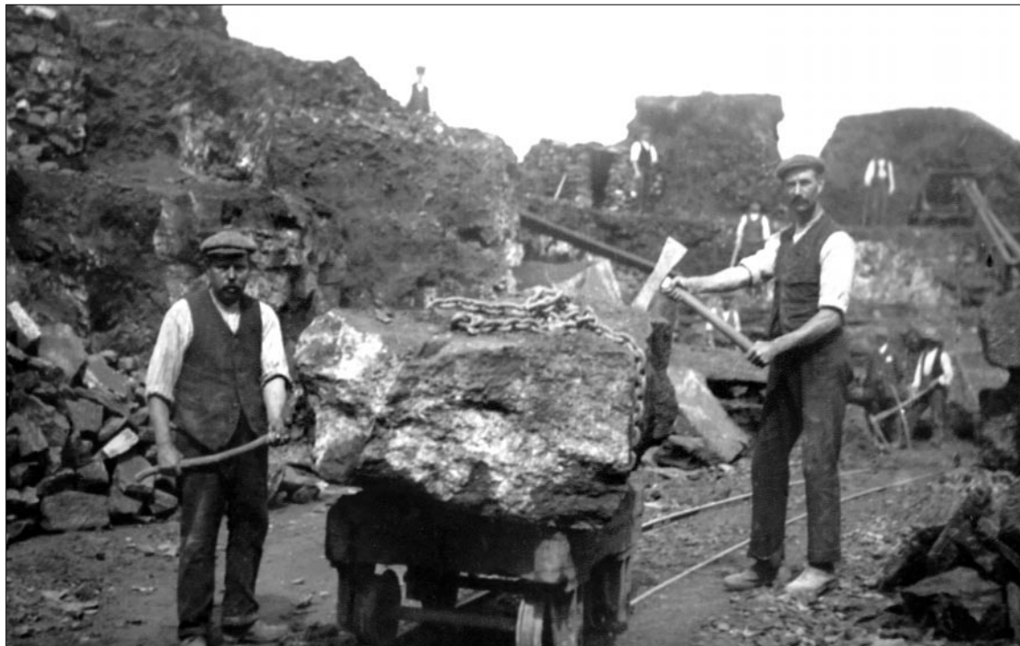
Stone being moved from the quarry by a trolley on rails, the easiest way to transport large stones to the quarry workshop. Up to the 1990s rails could still be seen at the site of old quarry workings.
